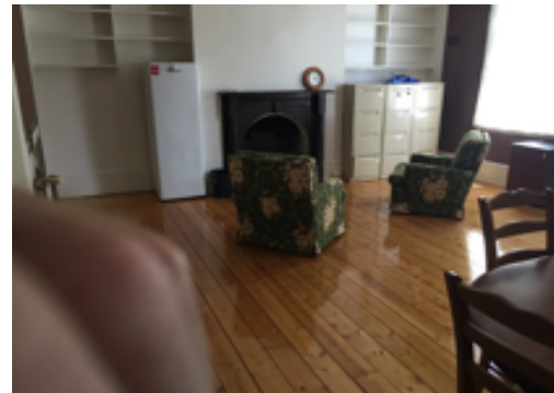
Room almost completed
