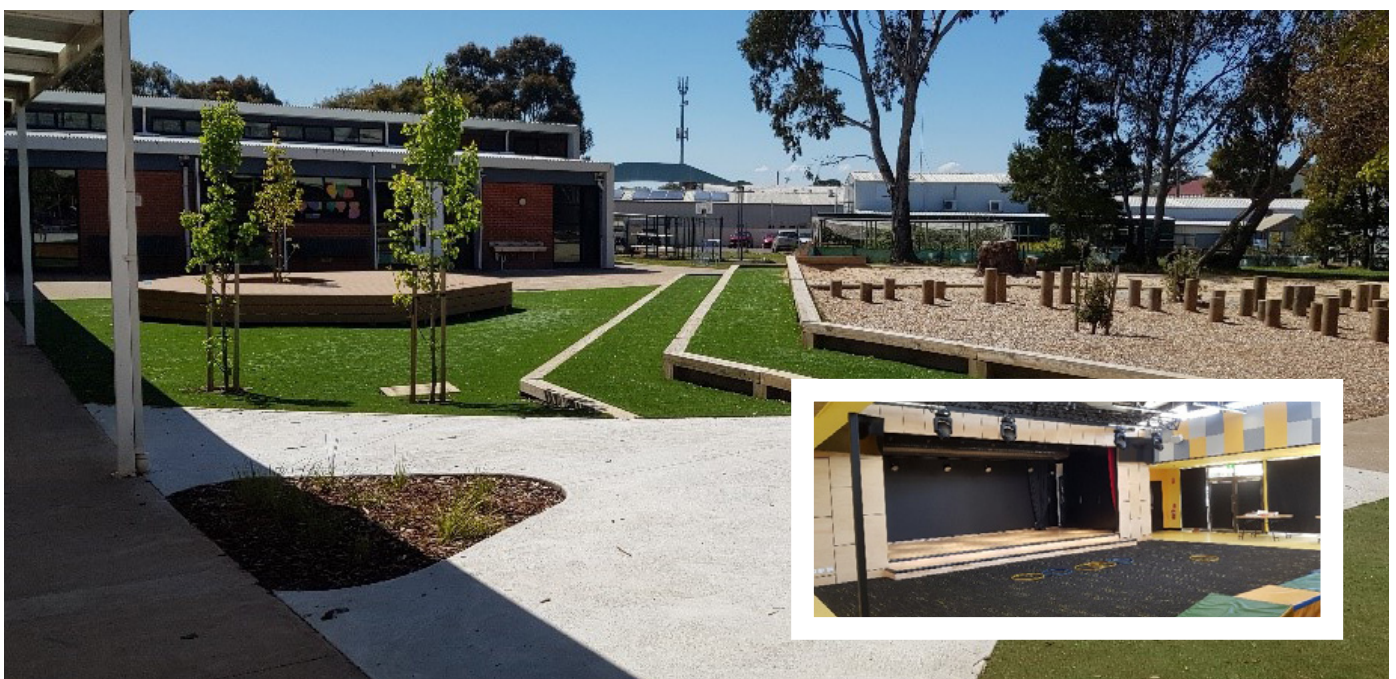
Extensive landscaping outside the Year 3 to 6 building and refurbishment of the student toilets in the prep and 1/2 areas have also been completed.
