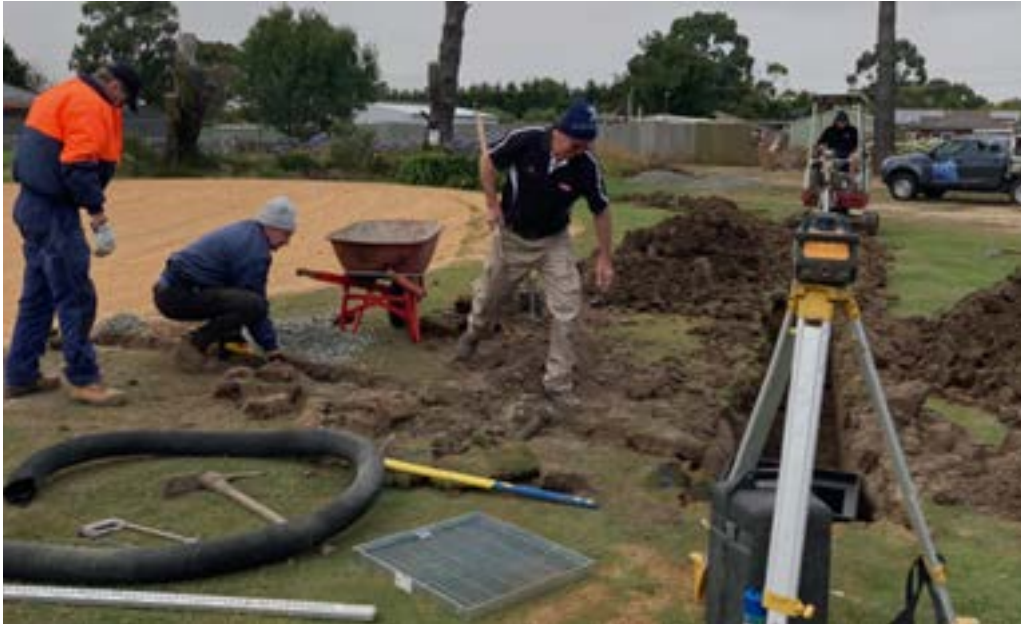
The team gets the drain at the 6th green moving.
