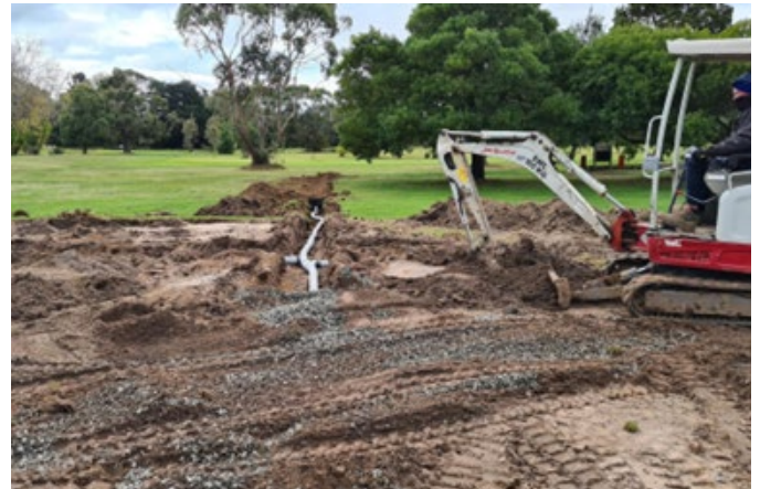
Mitch sorts the drainage on the new green.
