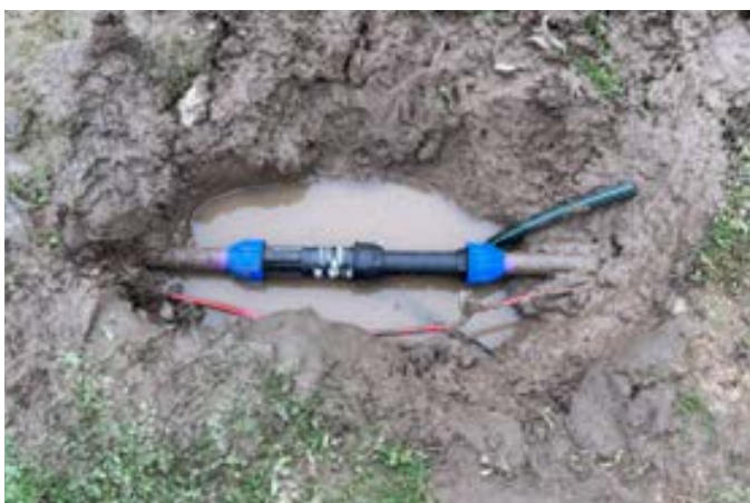
Leak repaired.
