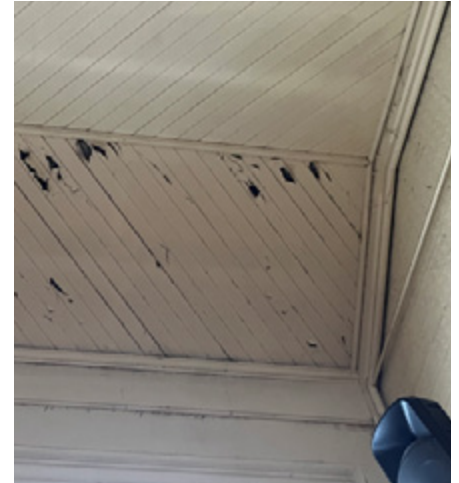
WATER damage to the ceiling
